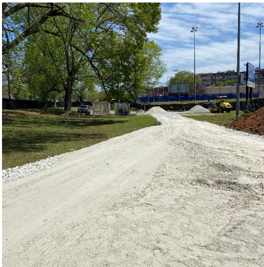
Access Road Aggregate in Place
