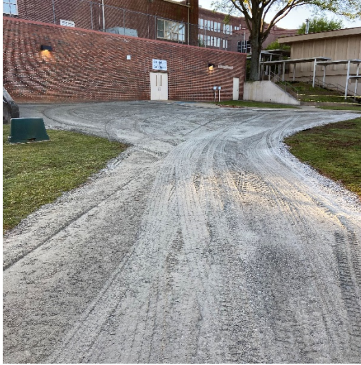
Crane Pad Installed
